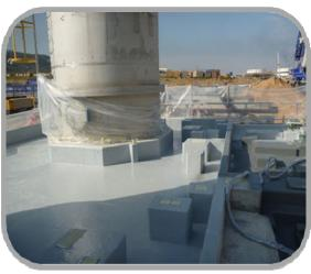
Ring beam protection, which is a common corrosion problem that occurs where a steel tank sits on a concrete base, was addressed with formal termination details submitted and approved by the Client.
