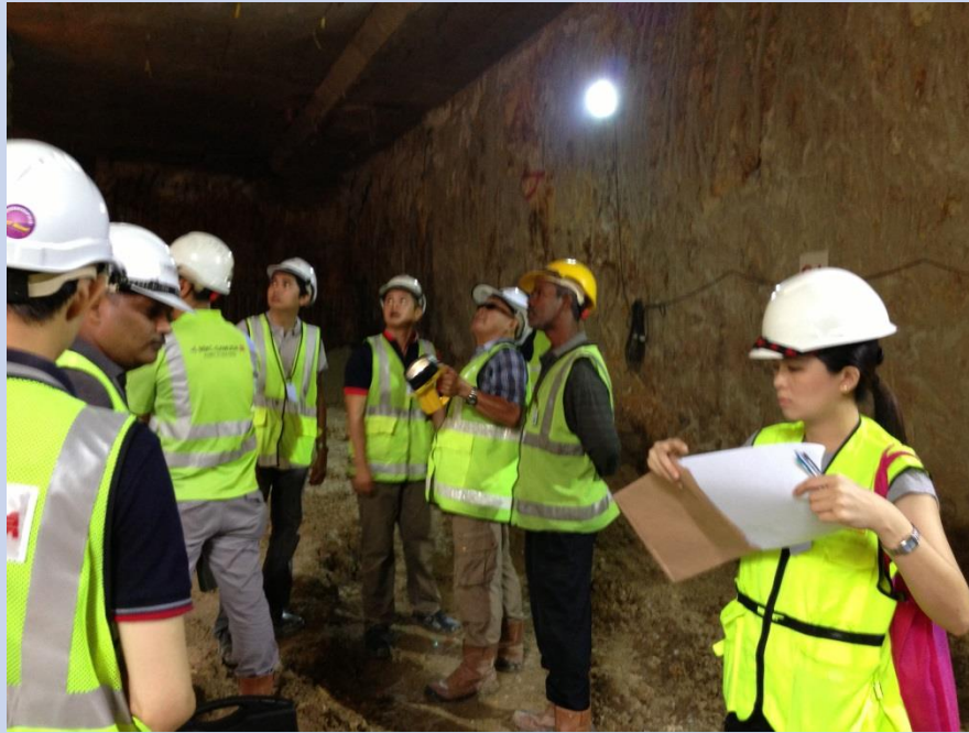
Inspection test with clients and consultant
