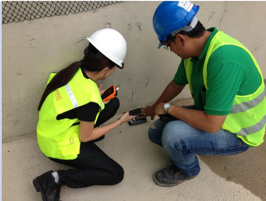
Moisture testing on concrete
