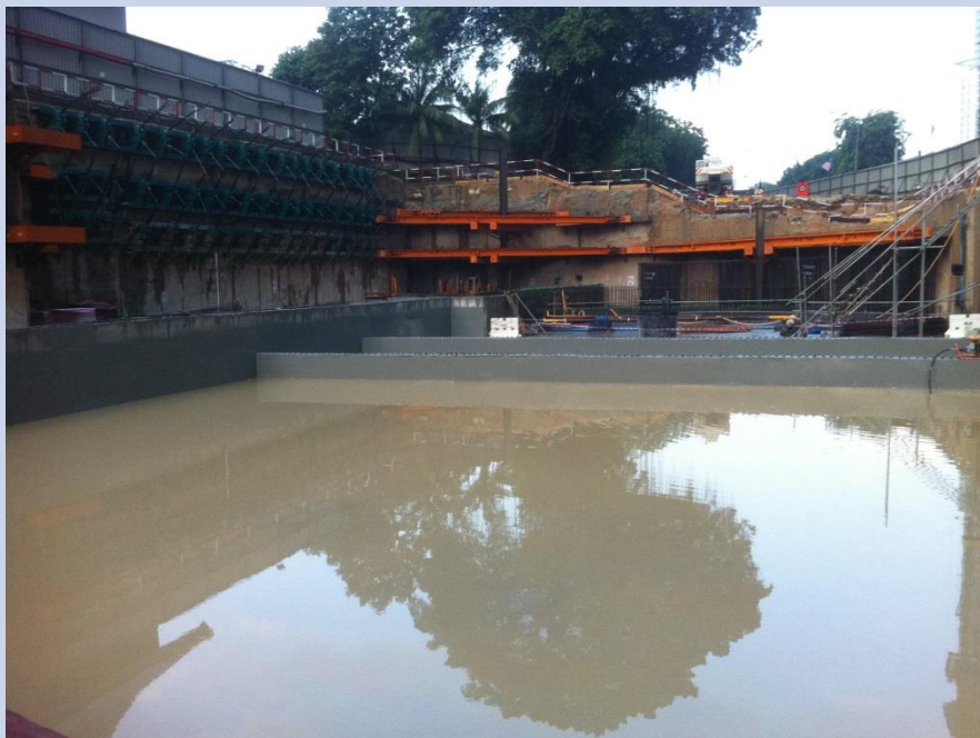
Water Ponding Test
