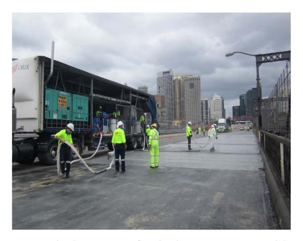
THE New South Wales State Government's Roads and Maritime Services commissioned this important maintenance project, which also included asphalt resurfacing. It was the first time in 80 years that the bridge deck road surface has been stripped back and waterproofing applied.
