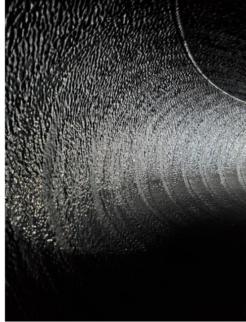
Liner Installed Bend 2
