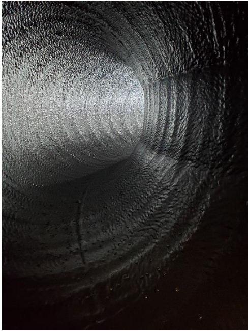
Liner Installed Bend 1
