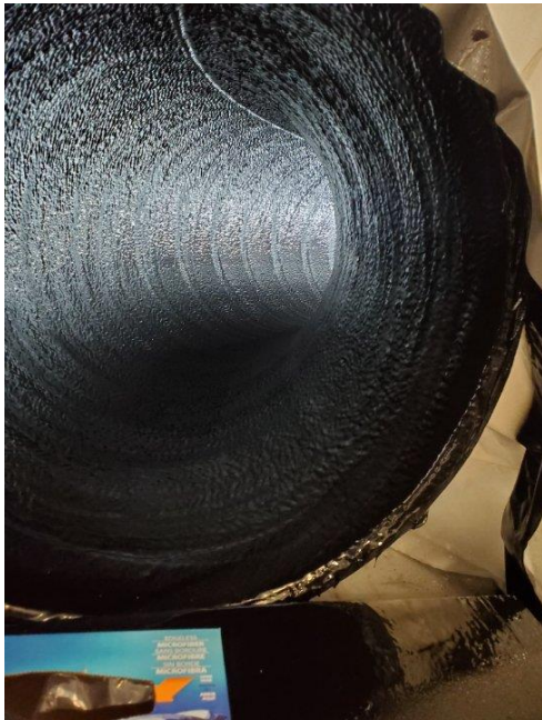
Liner Installed Bend 2
