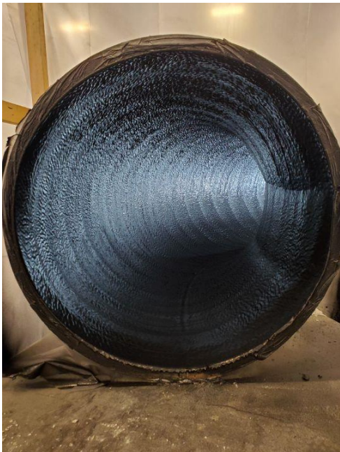
Liner Installed Bend 1
